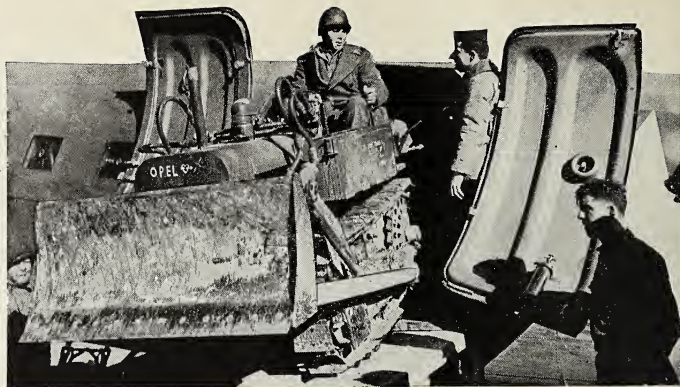
Unloading a bulldozer from a transport.
